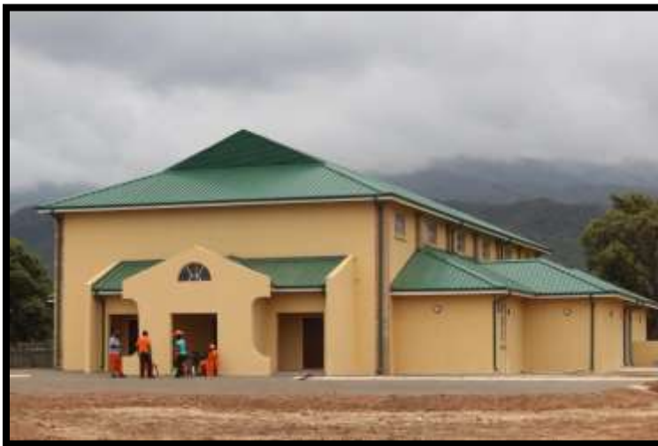
Moshate Community Hall
